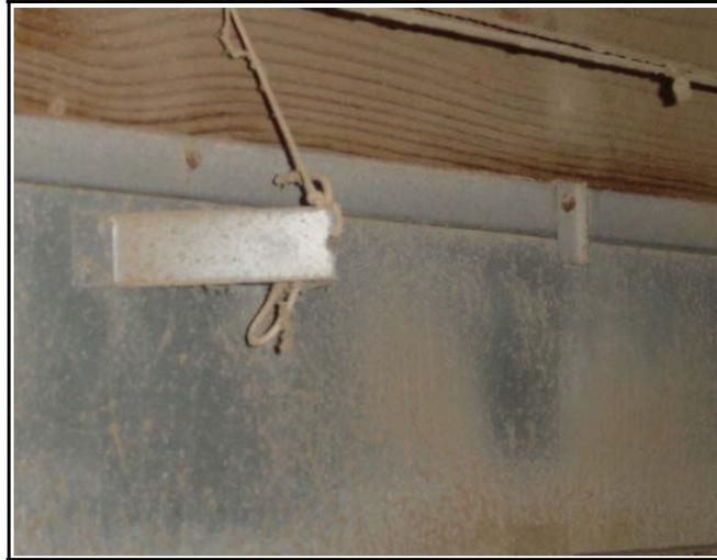
Figure 9. Air inlet latched closed.
